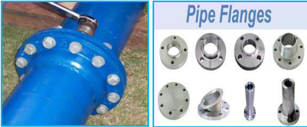
Fig: Flanged Joint of DI Pipe
