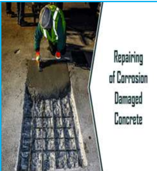
Rectification Concrete crack due to embedded reinforcement by additional concreting and cathodic protection
