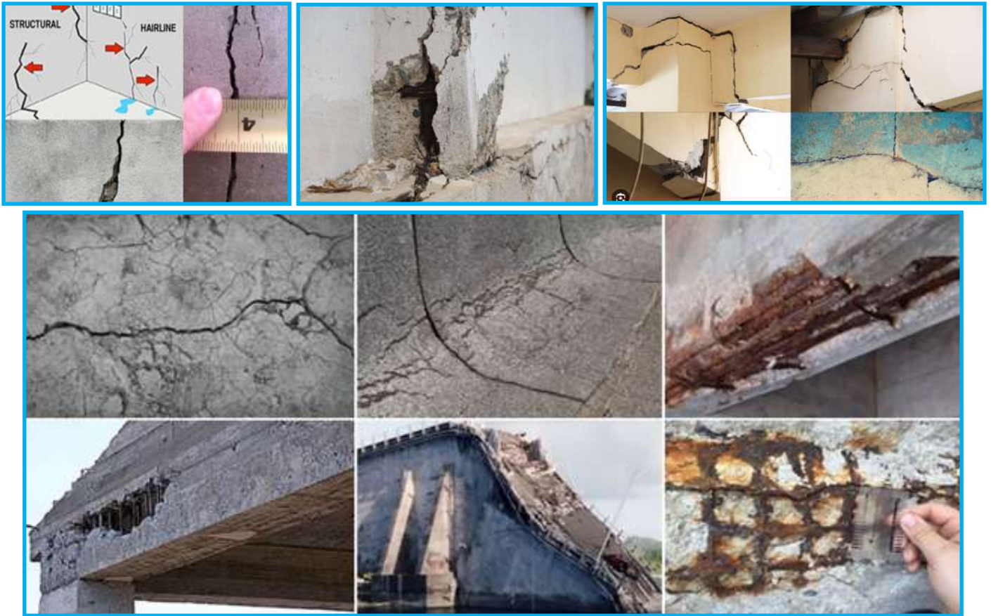
Structural Cracks in concrete
