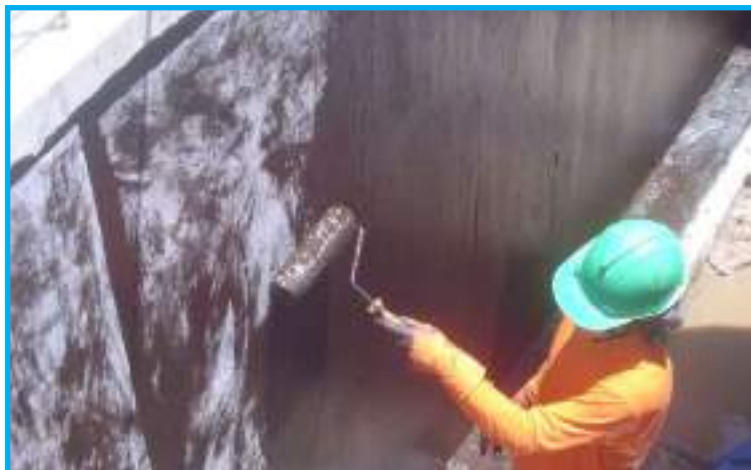
Underground Reservoir With Water Leaking From A Crack
