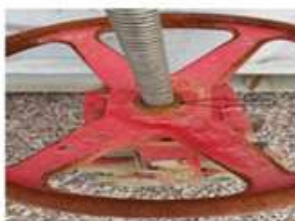
11 : Corrosion of stem nut may increase operating torque
