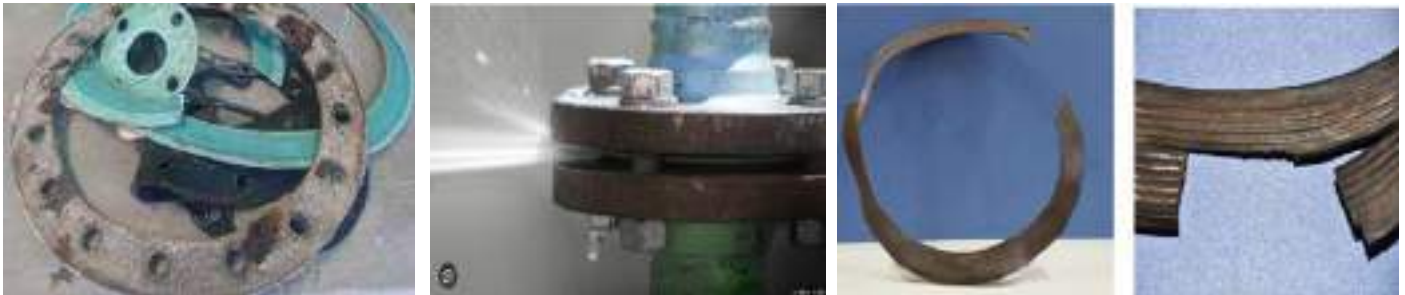
Fig: Damage of Flanges and Gaskets of a Pump
