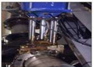
10 : Gland leakage in a valve in hot molasses line
