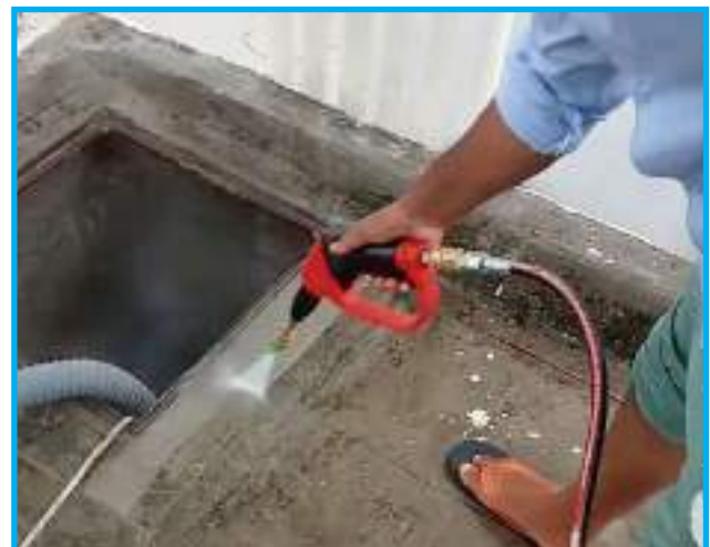
Repair, test and monitor
