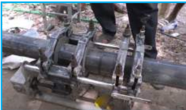
Installation of new joint with machine
