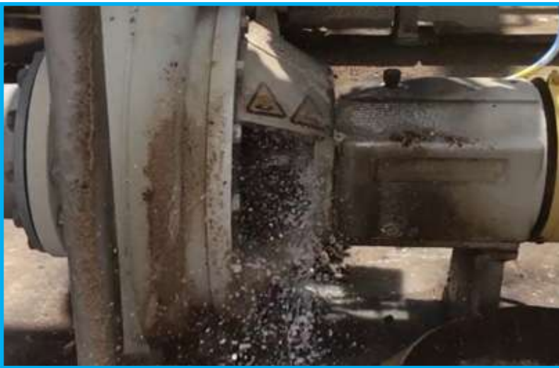
Fig: Damage of Mechanical seal of submersible pump
