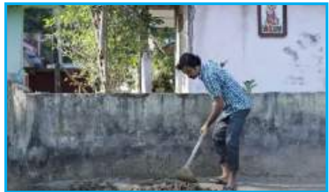
Excavation and Expose of Pipe Joint
