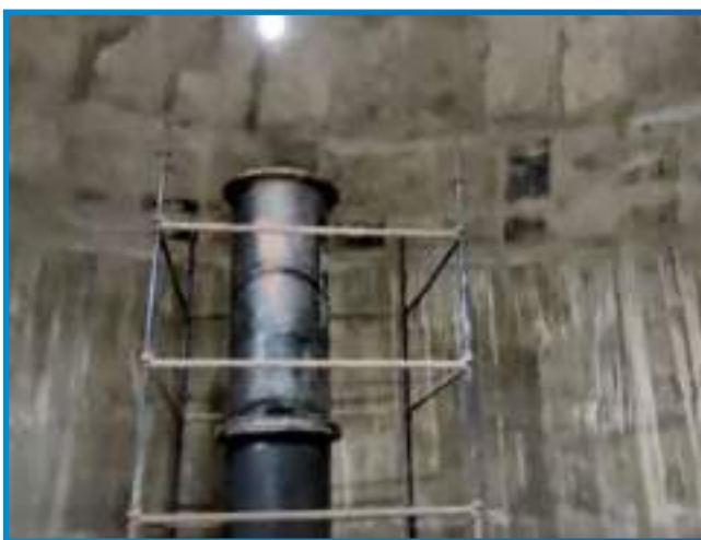
Inspection of blockage
