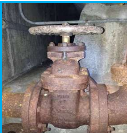
10 : Gland leakage in a valve in hot molasses line
