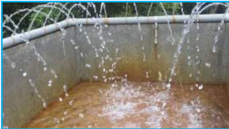
Clogged aerator with reduced water flow
