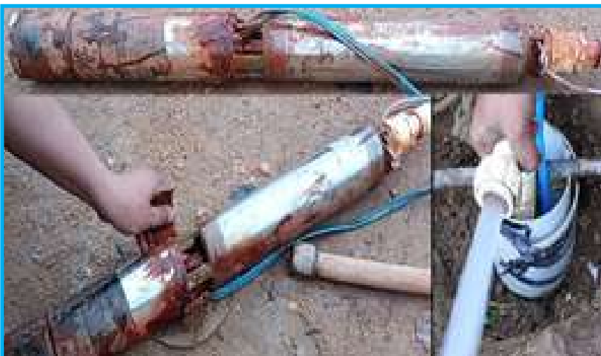
Fig: Repairing of Pump shaft of submersible pump
