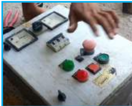
Component replacement from starter box
