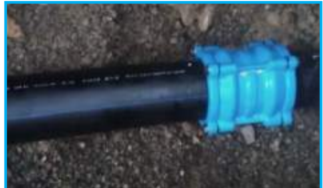
Connection of new joint
